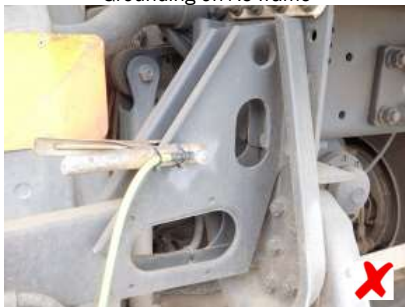
Grounding on AC frame
