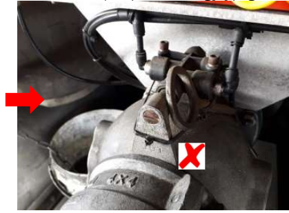
Unauthorized valve locking
