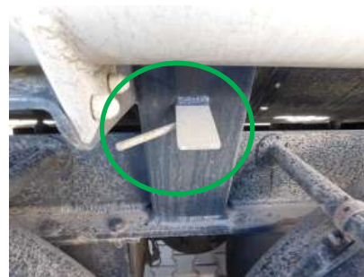
AC grounding point
