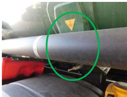
AC grounding point
