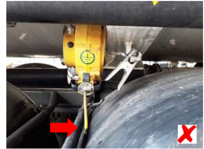
Earthing drum not working
