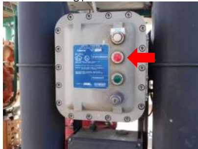
CIVACON not connected
